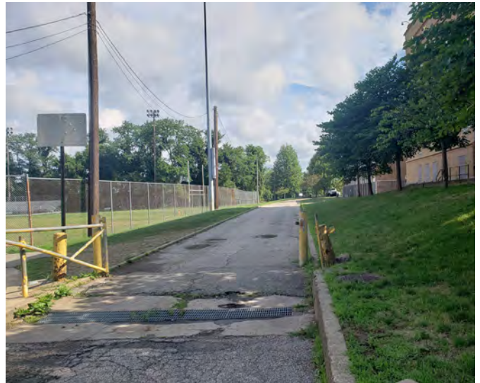
Existing roadway is in poor condition and narrow width does not allow for two-way traffic
