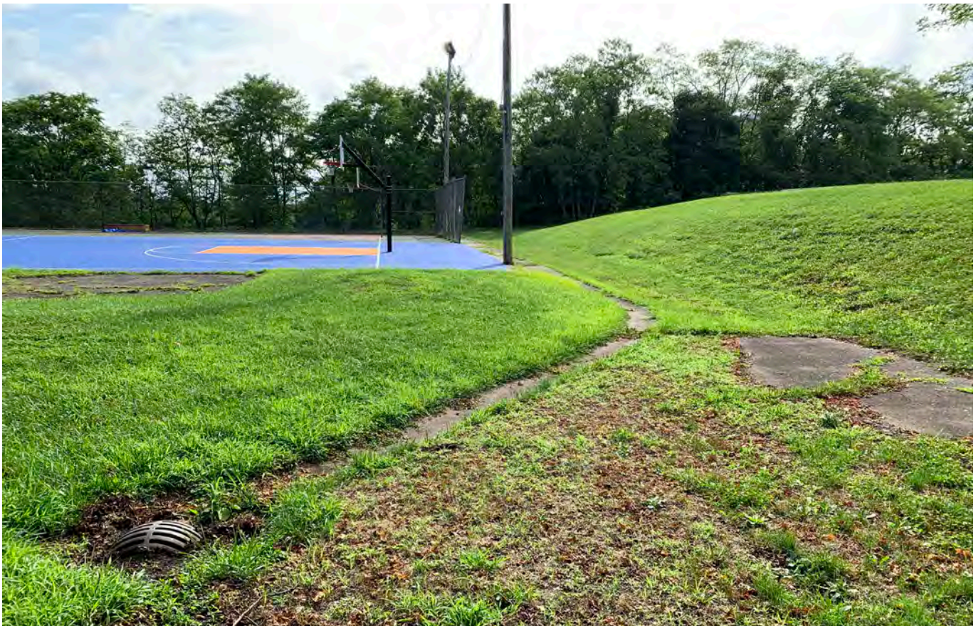
Existing drainage infrastructure is inadequate. Surface inlet can be converted to be the overflow within a new vegetated rain garden
