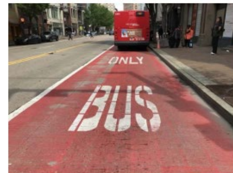
Dedicated bus lanes, such as this one on Liberty Avenue, separate buses from traffic and are especially beneficial at rush hour. Bright red paint helps the bus lanes stand out even more.
