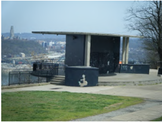
Photo 7 Grandview Park Bandstand. The bandstand is heavily covered in graffiti and should be repainted.
