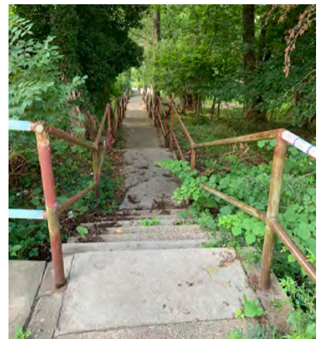
Existing steps from Hillcrest Street to Rosetta Street need new handrails and selective clearing on either side
