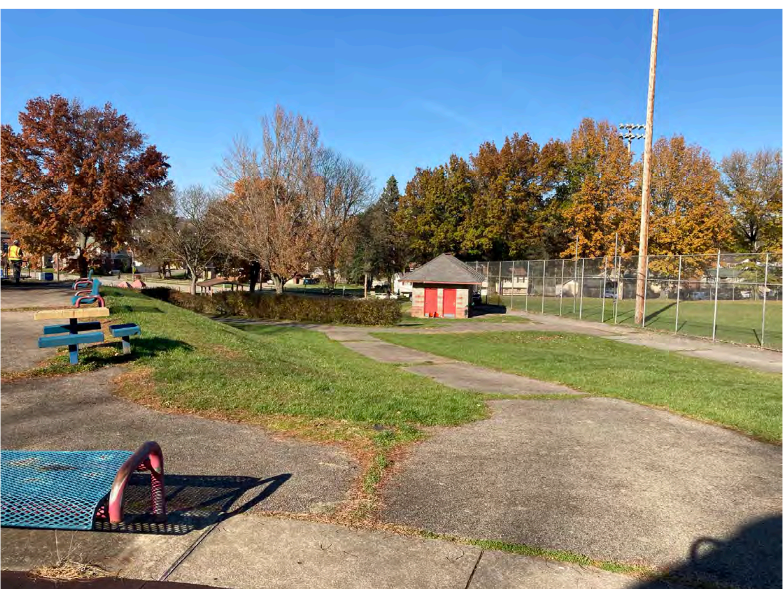
AGING & CRACKING ASPHALT
