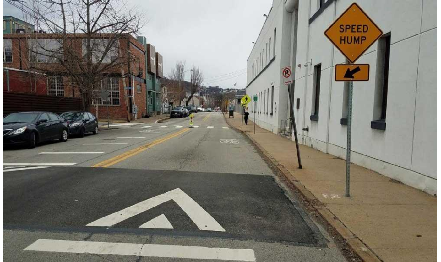
A speed hump installed as part of a Neighborway in the South Side
