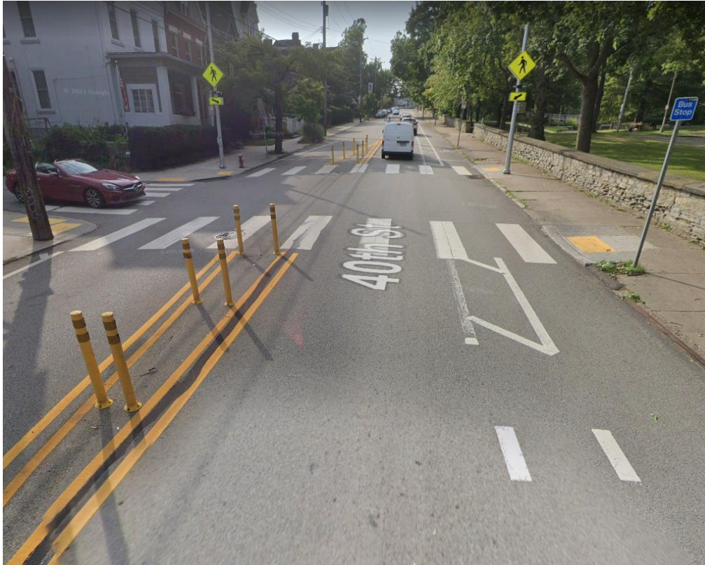
Pedestrian refuge island installed on 40th Street
