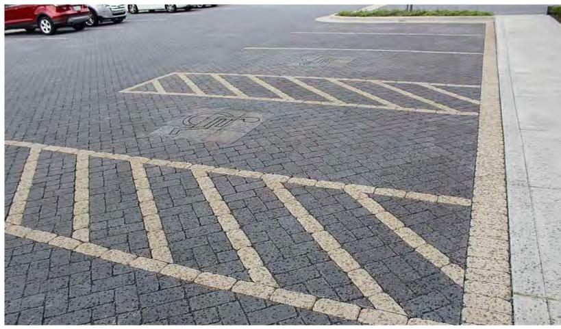
Pervious Paving - Parking Lot with Pervious Pavers
