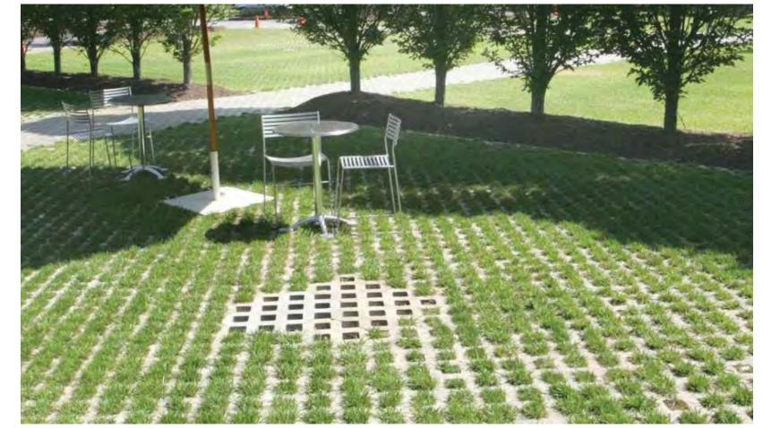
Pervious Paving - Concrete Grid Pavers
