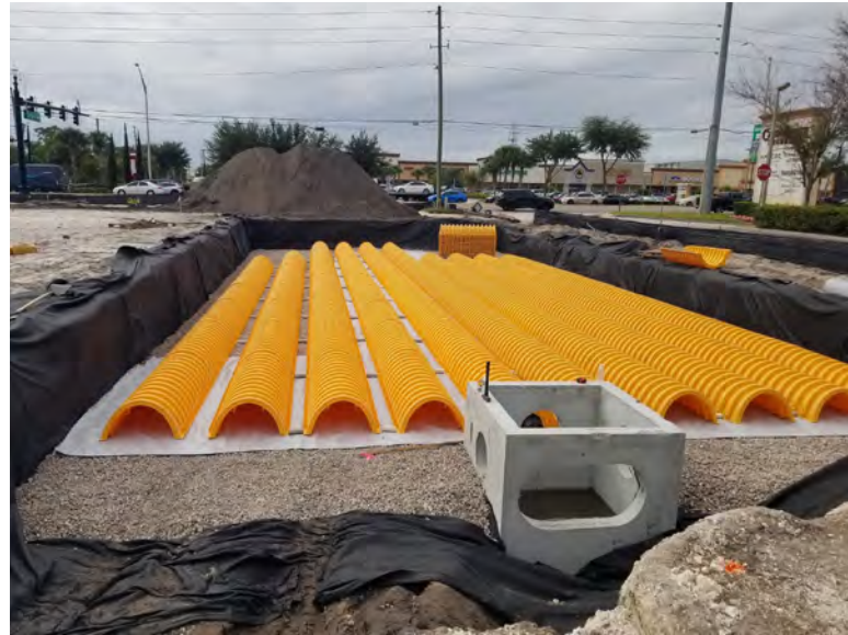
Subsurface Stormwater Storage Chambers
