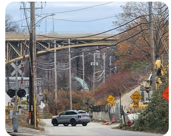
Electric lines along Neville Ave
